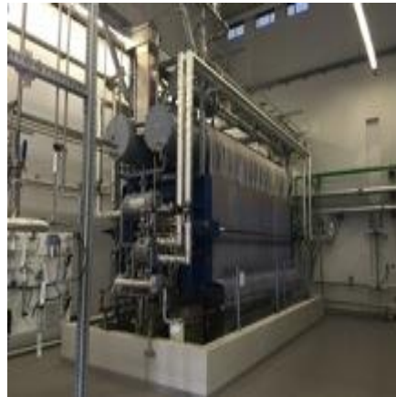
Production of hydrogen in 6 MW electrolysis
