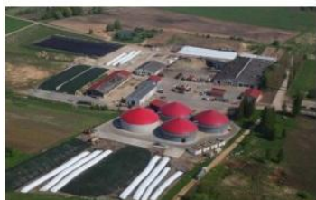
"Agroiecava" Ltd. Biogas plant produce heat for local municipality.
