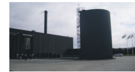
The district heating system in Sønder Omme in central Jutland uses wood chips, sourced in the surrounding forests to provide heating for 760 households as well as energy for surrounding industries.
