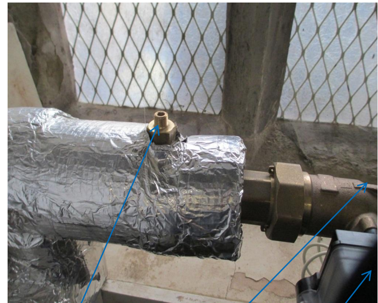
Temperature sensor connection point
